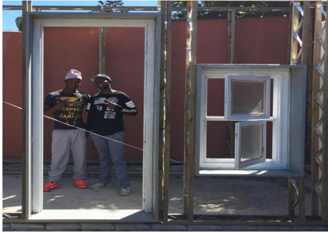
Figure 22: Window and door installation
