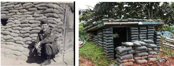
Figure 3: Sand-filled bags military bunker (Leiden 2011)
