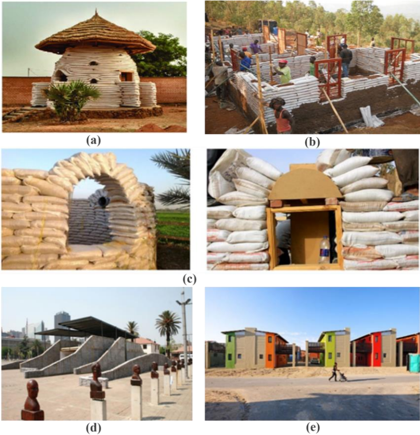
Figure 8: Houses constructed using sandbag technologies in Africa
