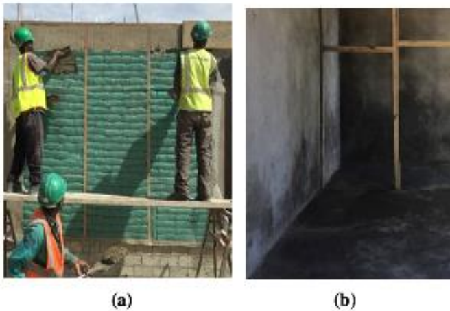
Figure 25: Wall plastering
