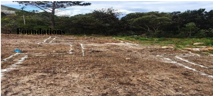
Figure 16: Sandbag site marking out
